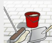
Sweep the paving surface with a soft broom until clear of all excess stone dust. The stone dust may leave a grayish residue which will wash off when it rains.
