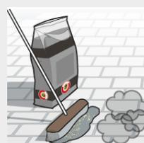
Sweep the filling materials into the joints using a soft broom. Sweep in a diagonal pattern until the joints are filled to the top.
