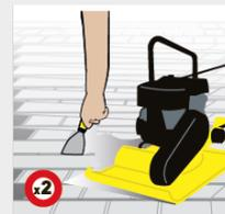
If the paving is new, vibrate twice using a protective rubber mat on the vibrating plate to avoid damage to the paving surface.
