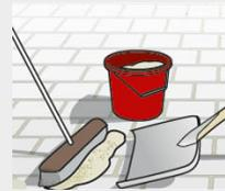
Sweep the paving surface with a soft broom until clear of all excess stone dust. The stone dust may leave a grayish residue which will wash off when it rains.
