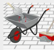
Mix the filling material in a bucket or a wheelbarrow using a shovel to mix the mineral additives with the silica sand. Never mix the contents from more than two bags at a time.
