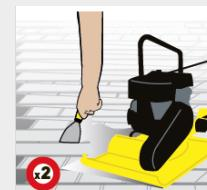
If the paving is new, vibrate twice using a protective rubber mat on the vibrating plate to avoid damage to the paving surface.
